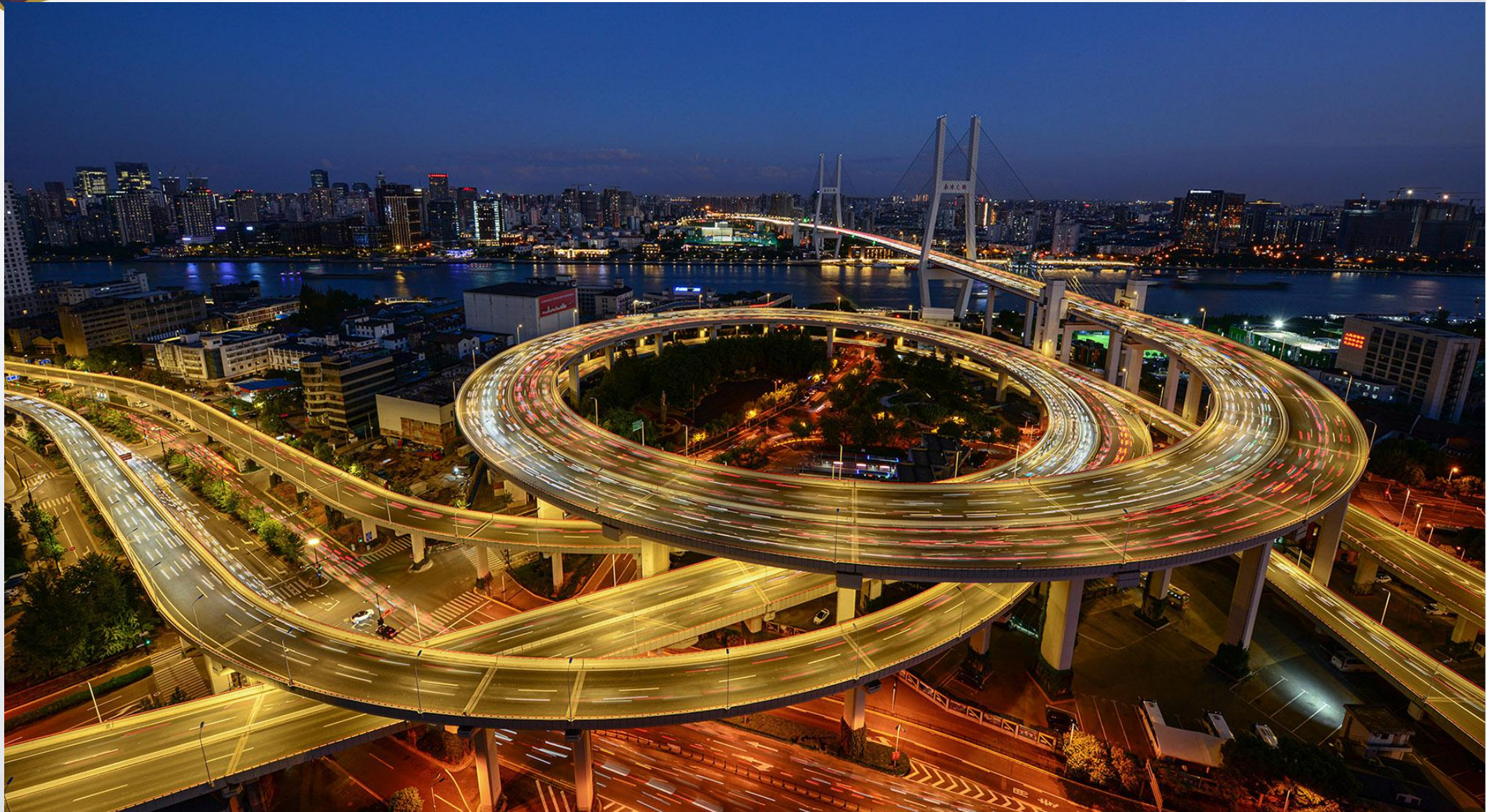
LAVASH MERIT E -CERTIFICATE | PHOTO TRAVEL (PTD)(DIGITAL) | NANPU BRIDGE 6 | ZHICAI REN | China
